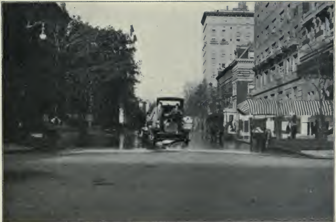
Motor-driven power flusher—Flushes entire width of street.
